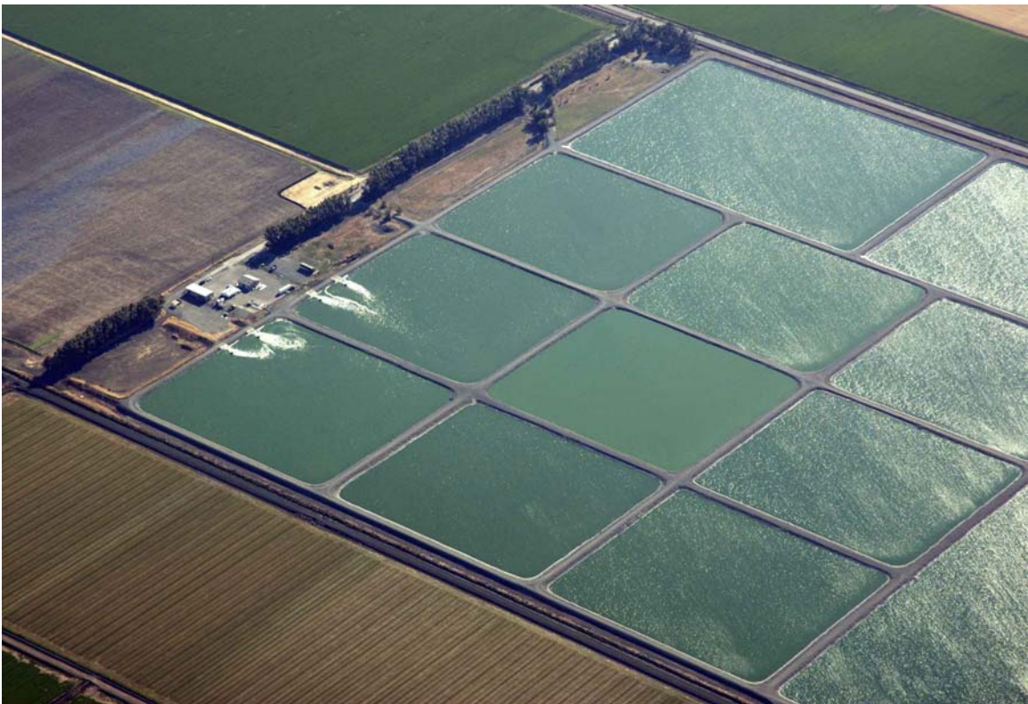
Figure 1: Aerial view of a portion of the Dixon Wastewater Treatment Plant
